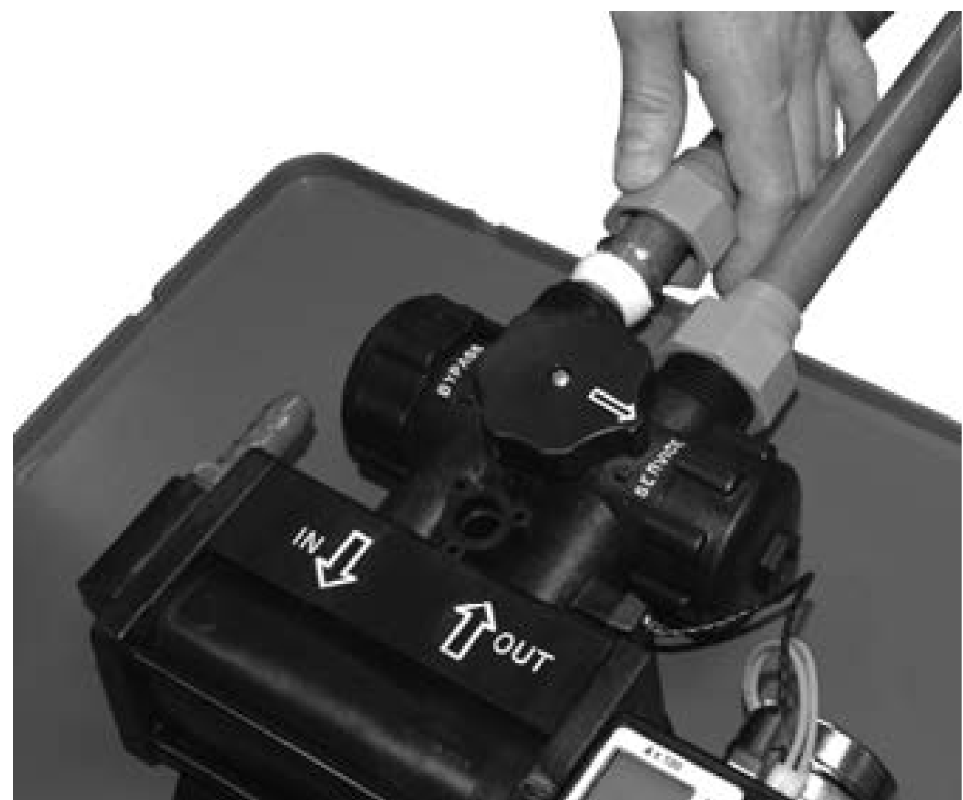
Figure 3: Connect Water Lines
